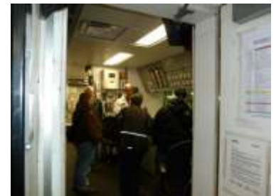
In the engine room office
